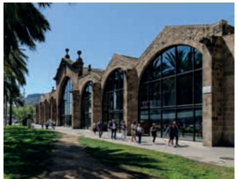
The facade of the Drassanes Reials
